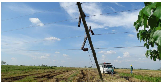
NGCP restored power flow through the Gamu-Roxas 69kV line which tripped due to a burned woodpole. Reports from the field indicate that the pole was affected by rice hay burned under the structure in Barculan, Gamu, Isabela.
